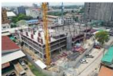
Fig 12: Kanjanasuk Carpark Building (Phranangklao Hospital) project
