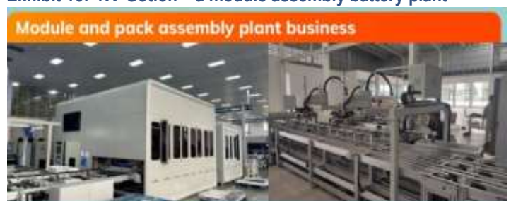
Exhibit 16: NV Gotion – a module assembly battery plant
